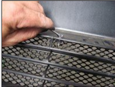
Picture #29: Fasten vent grille in place using supplied hardware.
